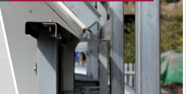
2 Folded gutter section – Water Management System
