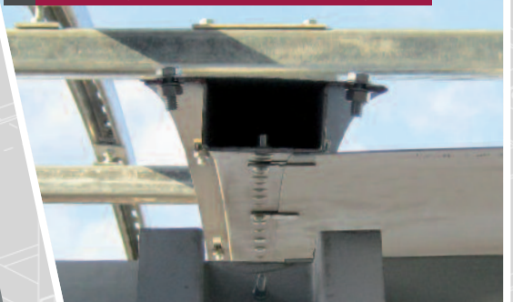
3 Rolled 'Top Hat' section to receive Polyvision
